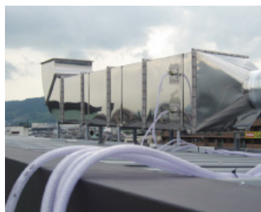
Spraying into an exhaust duct.
