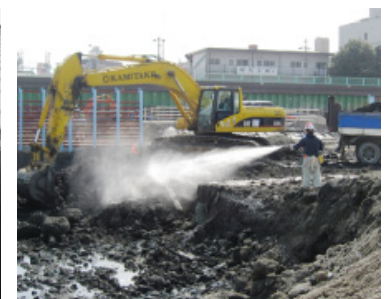
Sprinkling directly on to the source of smell.
